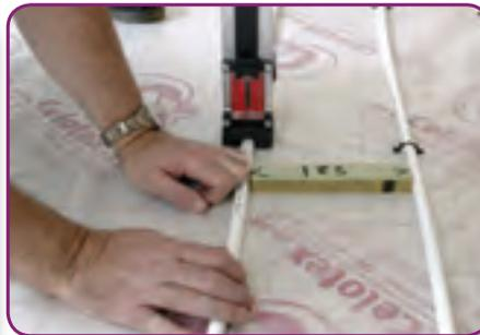
**STEP 5.** When using the pipe, unroll it from the outside of the coil and do not try to uncoil it from the centre, this will make the process easier. Keeping the first run of pipe around the perimeter straight and using a gauge to keep the designed pipe centres even will also help the installation process.
