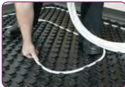
**STEP 5.** Starting from a manifold, after establishing the area to be covered, unroll the pipe and push firmly into the gap between the egg box sections. Cover the designed area in the appropriate pattern and return the pipework to the manifold.
