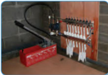
**STEP 4.** Connect a suitable pressure testing kit to one of the fill valves. With the valve open, pump up the pressure to 2 Bar. Isolate the pressure at the tester and leave for 10mins while checking for leaks or pressure drops.
