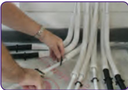
**STEP 4.** Run the pipework from the manifold to the room that is to be heated. Ensure that if the pipework is passing through other rooms that conduit is used to prevent the pipework influencing the heat in those rooms. Ensure the pipework is at least 75mm from the perimeter wall.
