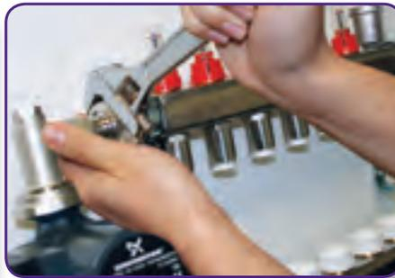
**STEP 2.** Using the supplied washer fit the JG control pack. Isolation valves fitted to the inlet side of this unit will be useful in the event of needing to change a pump or blending unit.
