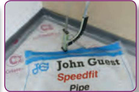
**STEP 3.** After establishing the area to be covered by the pipe circuit, connect to the manifold and start the circuit. If the circuit has to pass through other heated zones before reaching the zone it is intended to heat, conduit may be required.
