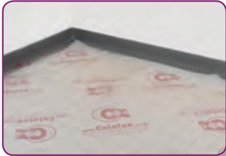
**STEP 1.** To prepare the floor, insulation should be fitted to a flat sub-base. The joints should also be taped and a membrane placed over the insulation.
