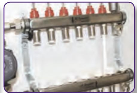
**STEP 3.** Connect the pipework to the manifold following the guidelines for fitting JG pipe and fitting. It is best to start from one end of the manifold and work to the other. The use of JG conduit elbows will make the process easier and neater and enable the conduit to be inserted into the socket end.
