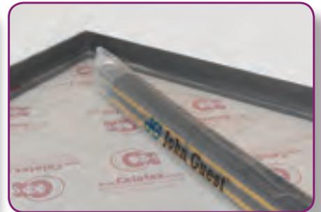
**STEP 3.** After establishing the area to be covered by the circuit, connect to the manifold and start the circuit. If the circuit has to pass through other heated zones before reaching the zone it is intended to heat, conduit may be required.
