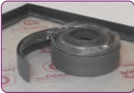
**STEP 1.** Edge insulation should be installed around the perimeter of the room to accommodate expansion that will occur when the screed is heated up. It is good practice to seal the gap between the potential space between the expansion and the floor panel.
