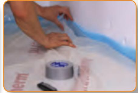
**STEP 3.** BS EN 1264 Part 4 requires a protective membrane placed over the insulation layer and it specifies Polyethylene film of at least 0.15mm thickness with 80mm overlaps or a similar product which performs the same function e.g. Aluminium Foil - fitted at the factory.
