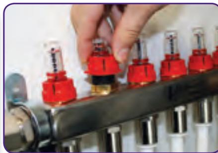
**STEP 5.** The flow meters at the top of the manifold give a visual indication of the amount of water flowing through each circuit. The amount of flow will depend on the length of circuit and the temperature drop required. Generally the shorter the circuit the more restriction will be needed; this is called balancing the system.
