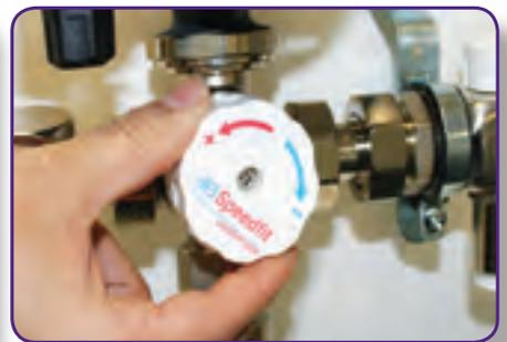
**STEP 6.** The designed temperature through the circuits is controlled by turning the blending valve knob to the desired temperature.
