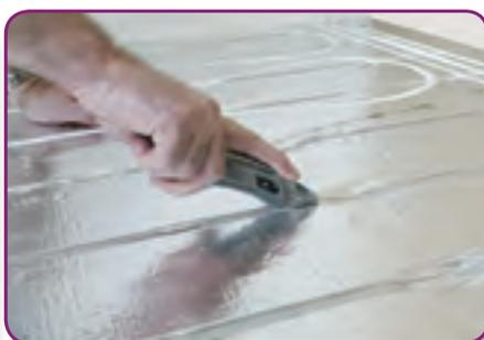
**STEP 5.** Where the pipe changes direction cut the foil in the return loops using a craft knife to prevent damage to the board. This will ensure a tight fit for the pipework.
