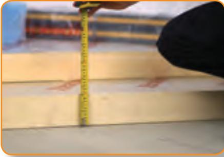
**STEP 1.** Insulation depth and quality as required by design or building regulations, “whichever is greater” and to ensure that any downward heat loss from the Underfloor Heating does not exceed 10W/m<sup>2</sup>, in accordance with BSEN1264.
