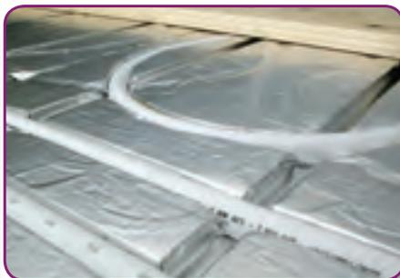
**STEP 2.** Plates need to be supported so that they sit level and make a good contact with the floor placed on them from above. Maintaining this contact is essential in producing good heat transfer.
