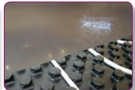
**STEP 6.** Once the pipe circuits have been installed and pressure tested, the system should remain under pressure (6 bar) in order to prevent the risk of any damage being caused to the pipe while the screed is being applied. When applying the screed cover, care should be taken to ensure that the screed is tightly compacted.
