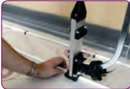
**STEP 4.** Using the staple gun, fix the pipework to the installation in the desired pattern (see page 15 images on patterns of pipework). Starting the first circuit 75mm from the perimeter and staples should be approximately 500mm apart. More staples maybe needed on bends.
