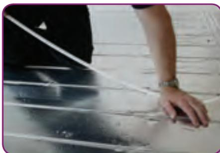
**STEP 4.** Start laying the pipework by pressing it firmly into the grooves. Where the pipework is connected to the manifold there will be a need to use plain insulation and pipe staples to accommodate the closer pipe centres.
