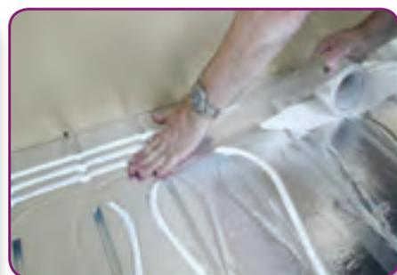
**STEP 6.** After installing the pipework JGTAPE can be placed over the end loops to prevent the pipework from becoming dislodged during the installation of the finished floor.
