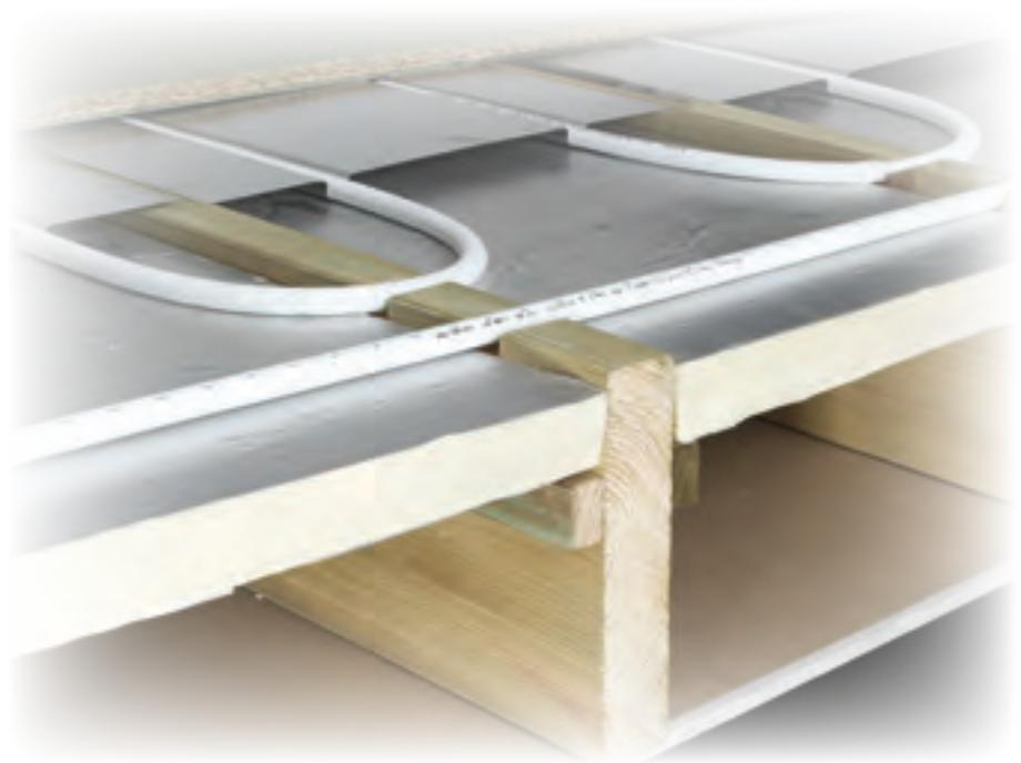
**STEP 1.** Plates need to be supported so that they sit level and make a good contact with the floor placed on them from above. Maintaining this contact is essential in producing good heat transfer.
