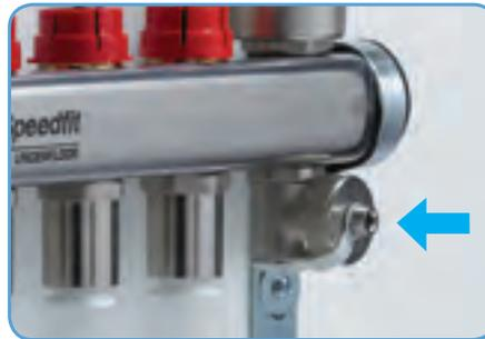
**STEP 5.** Connect the fill hose to the top hose connector valve on the manifold Flow Rail. Ensure the valve is in the open position.
