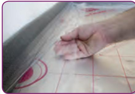
**STEP 2.** An expansion strip is required around the perimeter of the room to accommodate the expansion which will occur within the screed as a result of heating up. This should be fitted around the perimeter of the room and taped to the membrane.
