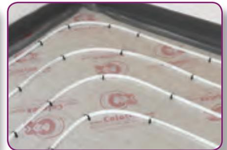
**STEP 6.** Once the pipe circuit has been installed and pressure tested, the system should remain under pressure (6 bar) in order to help prevent the risk of any damage to the pipe while the screed is being applied. When applying the screed, care should be taken to ensure the screed is tightly compacted around the pipe ensuring no voids are present.
