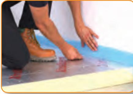
**STEP 2.** An expansion strip is required to accommodate the expansion which will occur within the screed as the result of it heating up. This expansion strip should be fitted round the perimeter of the room and taped to the membrane.
