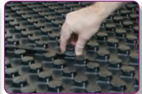
**STEP 3.** The "egg box" sections of the panel clip firmly together to make a continuous seal. Floor panels should not be used at the base of a manifold as pipes need to be closer together than the floor panels will allow. Pipes around this area should be secured using pipe staples.
