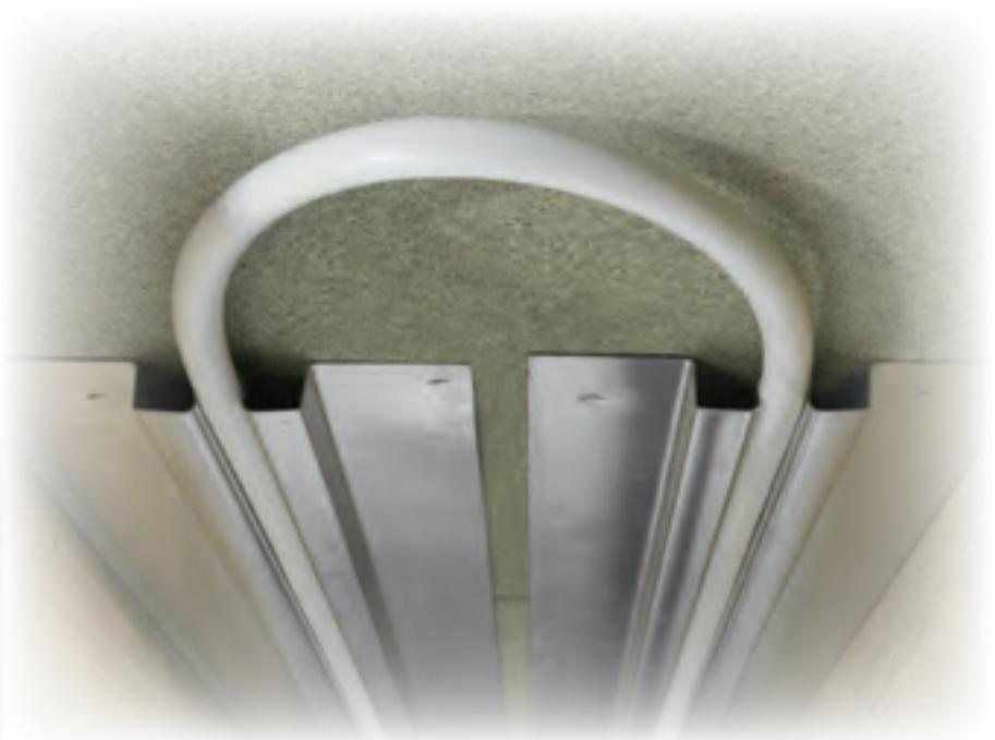
**STEP 1.** Planning is important to establish the areas that are to be fitted with plates and the route the pipework must take from the manifold to the area to be heated. Remember that the pipework can pass through the joists in the same way that the Heating and hot and cold pipes do. Make sure that any drilling zones are observed.
