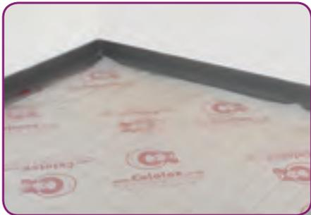
**STEP 1.** To prepare the floor, insulation should be fitted to a flat sub-base. The joints should be taped and membrane placed over the insulation.
