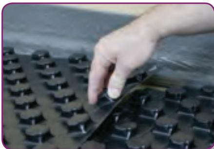
**STEP 4.** When a pumped (liquid) screed is to be used it is essential that all of the panel joints are made correctly and that no panels are allowed to simply 'butt-up' as this may allow the screed to flow below the panels causing them to rise up.
