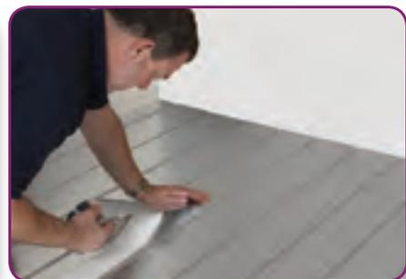
**STEP 3.** After placing the boards and ensuring they are flat and level and the joints are butted up firmly. Tape the joints using JGTAPE.
