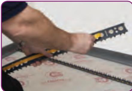
**STEP 4.** The mounting rail has double sided tape, this may need to be supplemented with the use of JGUFHPIN depending on the adhesions of the installation.
