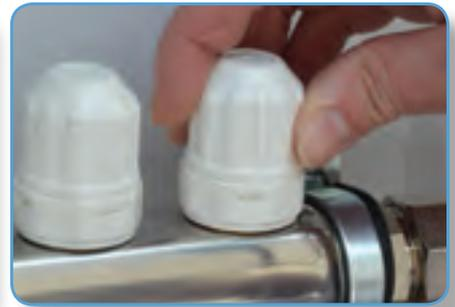
**STEP 3.** Ensure all Temporary Adjuster Heads are in the open position by turning the Adjustor Heads anti-clockwise.
