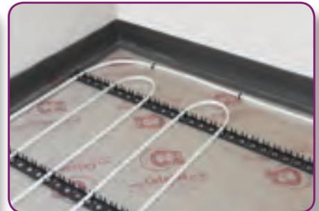
**STEP 6.** A serpentine pattern is usually the most convenient to use with the mounting rail system. Ensure to allow enough space at the end of the circuits for the flow and return from the manifolds.
