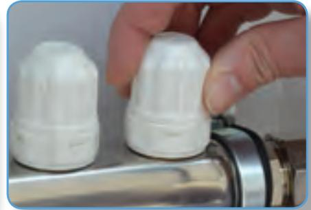
**STEP 3.** Ensure all Temporary Adjuster Heads are in the closed position by turning clockwise.
