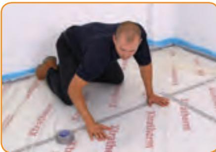
**STEP 4.** This vapour barrier will prevent the contamination of the insulation by the screed. It will also prevent liquid type screeds from flowing between gaps in the insulation and “floating” the boards during installation.
