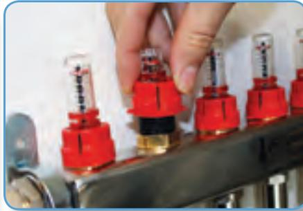
**STEP 2.** Open all flow gauges at the top of the manifold by lifting the locking cover and turning the adjuster anti-clockwise.
