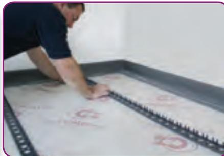
**STEP 5.** The mounting rail is placed at about 750/800mm apart ensuring the slots are aligned neatly.
