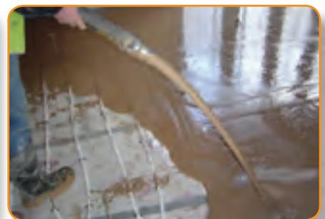
**STEP 6.** Screed depths need to be taken into consideration as part of the floor build thickness. (See page 20 for typical floor section).
