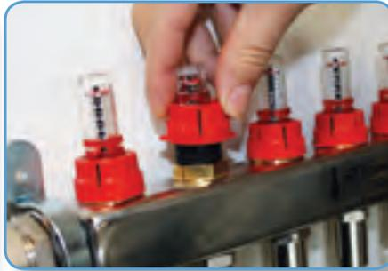
**STEP 2.** Open all flow gauges at the top of the manifold by lifting the locking cover and turn the adjuster anti-clockwise.
