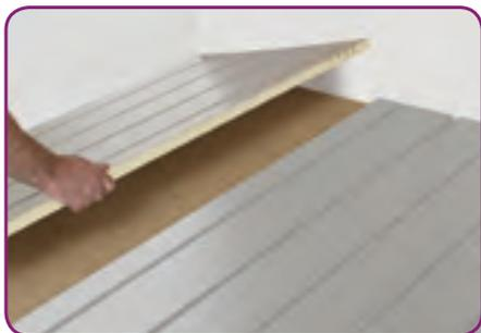
**STEP 1.** The main consideration is the amount of runs and the route those pipes will take from the manifold. If more transit grooves are needed then the grooves at the opposite ends can be cut off and used. Where possible route pipes through rather than around walls and doorways to cut down on pipework congestion. When lining up panels use a short length of pipe placed in the grooves to align them together.
