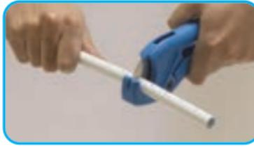
Make sure the pipe is cut square and remove burrs and sharp edges as these will damage the rubber 'O' ring. Always use a pipe cutter rather than a hacksaw.
