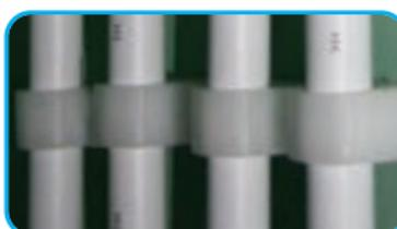
Pipe Clips should not be fitted any closer than 60mm from the end of the fitting. Pipe should be adequately supported by the use of Pipe Clips to prevent any undue stress.
